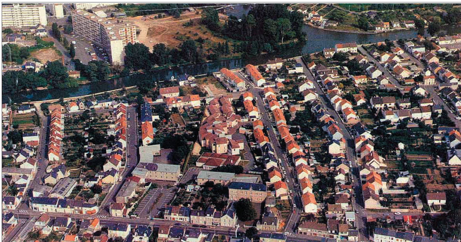
Quartier Olivier Heuzé (photo Services Techniques CUM)
