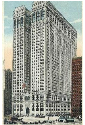
The Equitable Building
